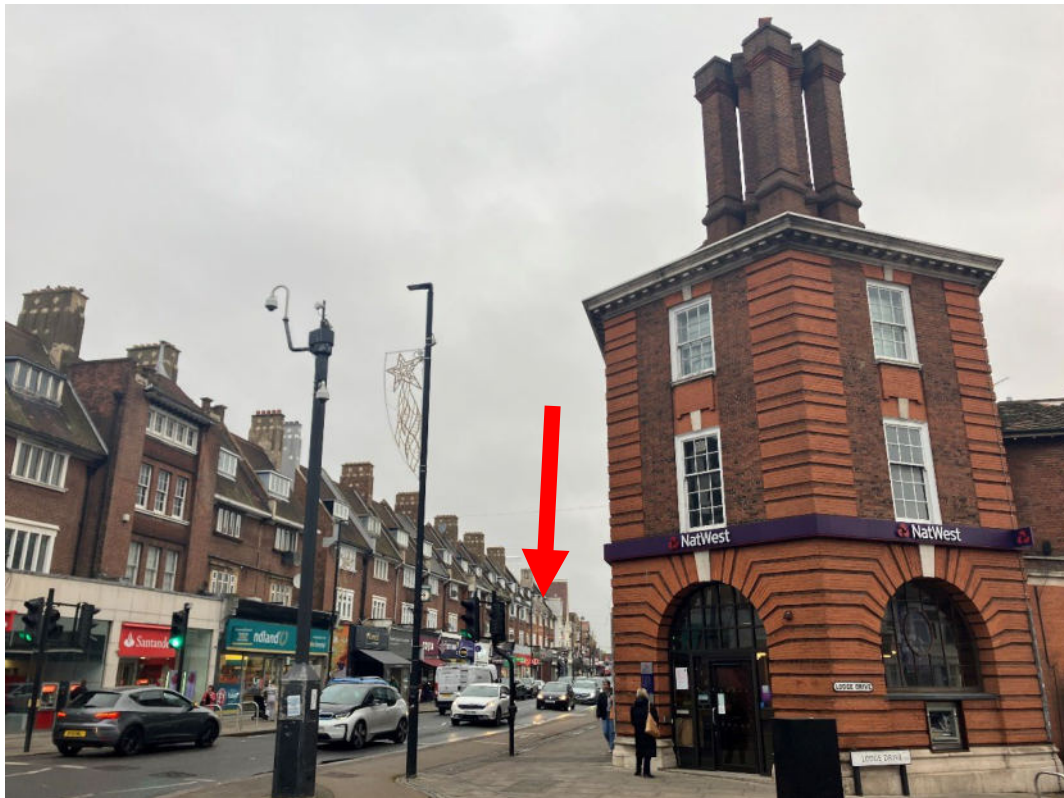
Plate 2: View north to Site (indicated) past Grade II National Westminster Bank.
