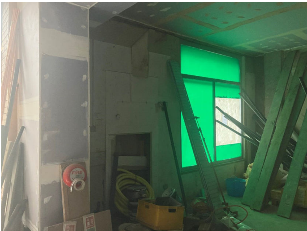
Plate 4: Interior view of Site shopfront.
