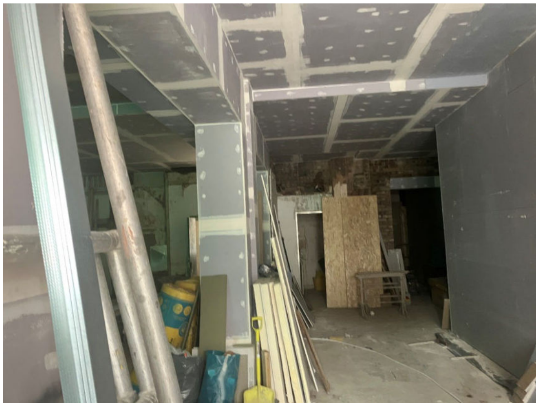
Plate 6: General Interior view of Site.
